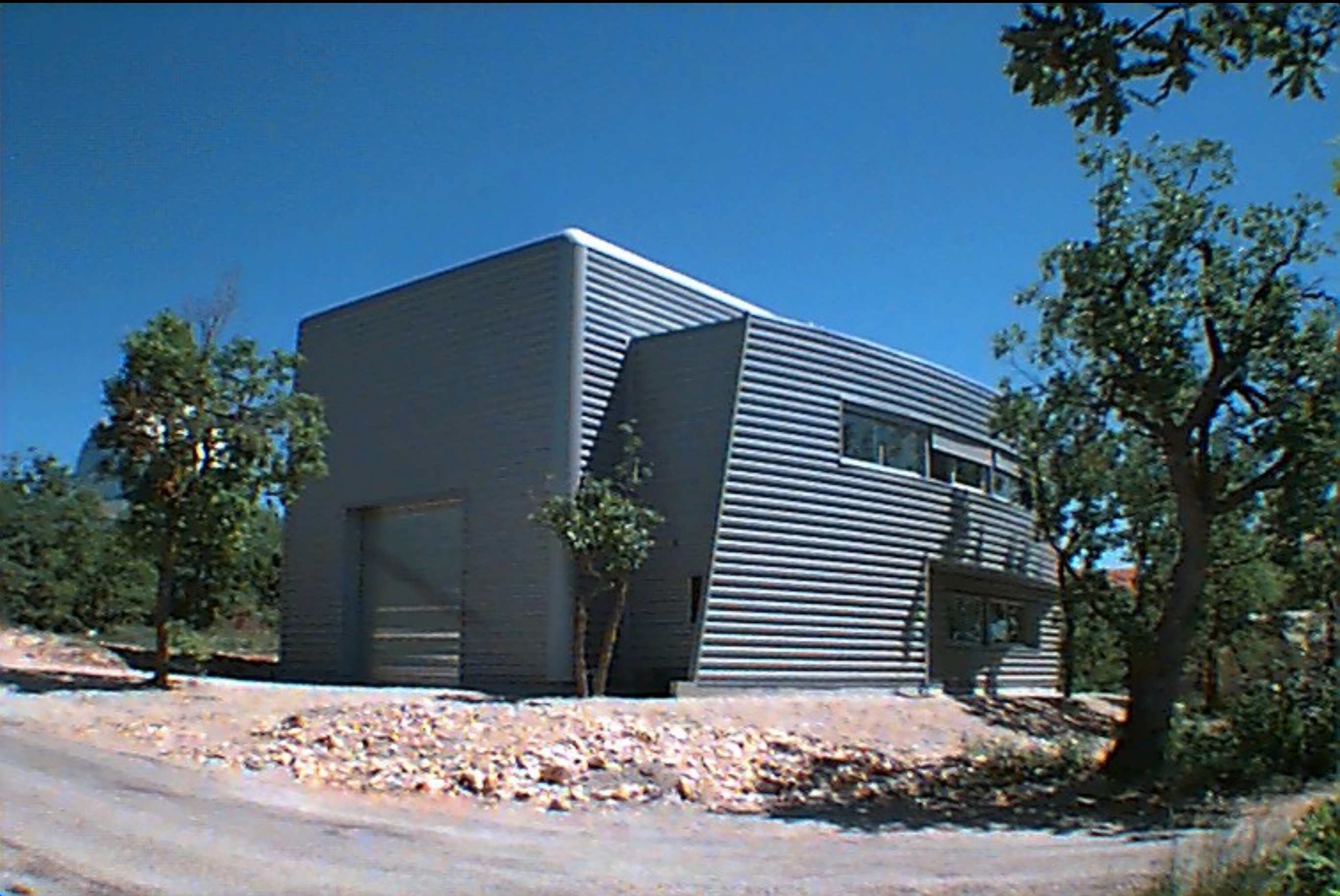
OHP Integration hall, built on purpose
